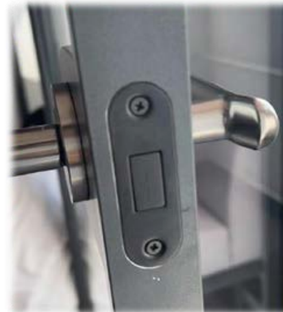
Magnetic Silent Door Lock (retracted)
